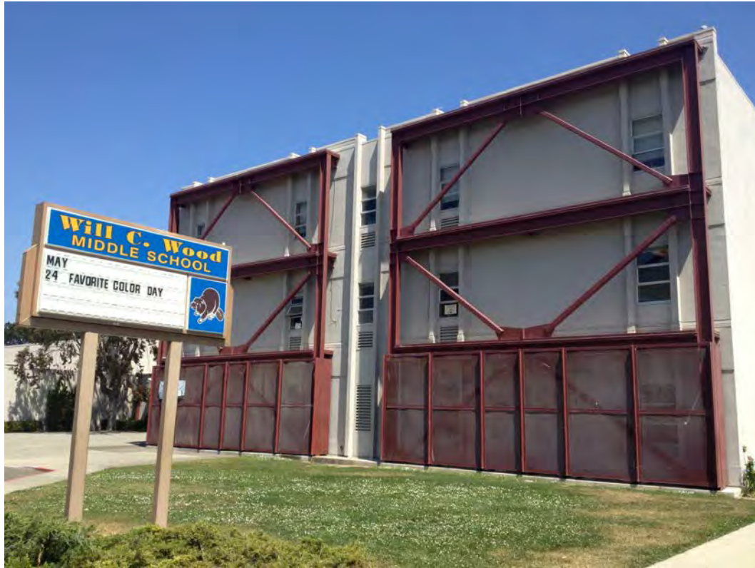
Seismic framing components at Wood Middle School (exterior installation)
